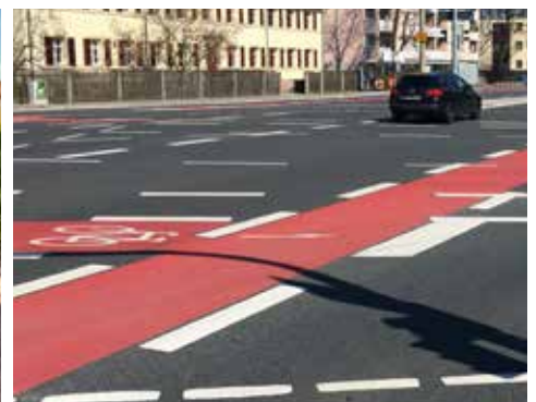
Red-coloured bicycle lanes: Layer thickness: 1-2mm - for heavy loads: 3mm. PlastiRoute + PREMARK symbols and arrows)
