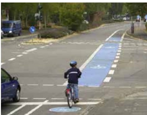
Bicycle area markings: 0.25 x 0.5m, line spacing 0.5:0.2m
